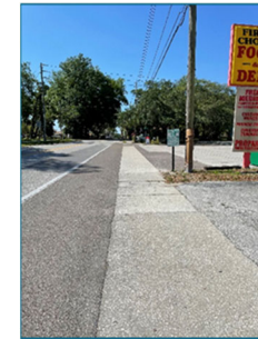
Figure 10: Sidewalk Lacking Separation from the Roadway Source: Kimley-Horn
