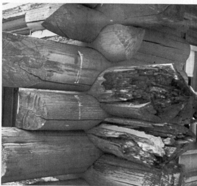
Fig. 19. Log splicing with scarf joints. Drawing: Harrison Goodall.
