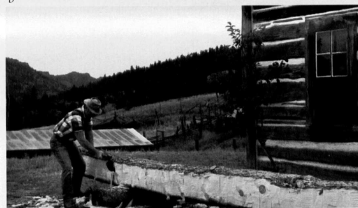
Fig. 11. Log-hewing tools and techniques: (a) scoring the log with a single-bladed felling axe, or "pole axe" in preparation for removing a uniform thickness of wood; (b) removal to depth of scoring; (c) finish hewing with a broad axe. Photos: Courtesy Bernard Weisgerber.
