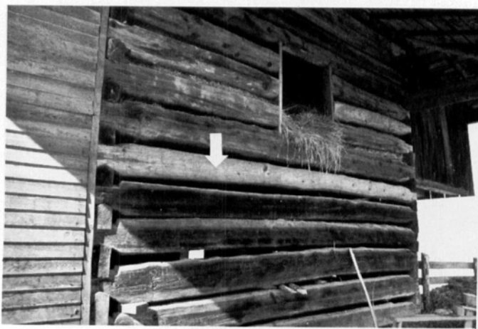
Fig. 22. The lighter-colored replacement log in this barn matches the dimensions and hewing marks of the original logs, and will darken in time to blend visually with the other logs. Photo: Bernard Weisgerber.
